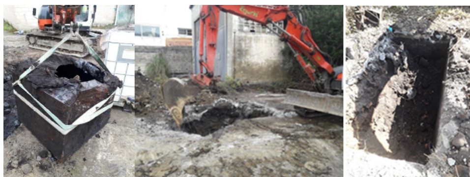
Figure 3. Image of fuel oil tank after digging it up and the excavation of the hydrocarbon-contaminated soil
