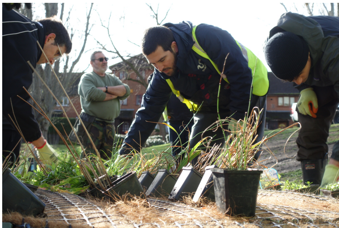
Figure 16: Volunteers laying out the plants into the coir matting and planting the wetland units.
