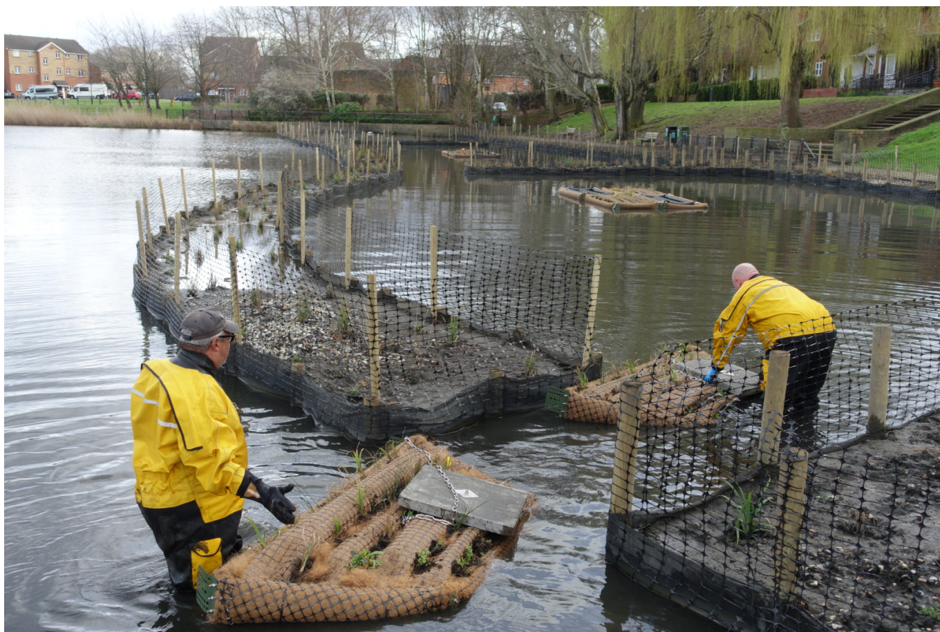
Figure 12: Concrete plates and anchoring chains being transported on the floating wetland units passing through the existing revetments at Gallions Lake, Thamesmead.
