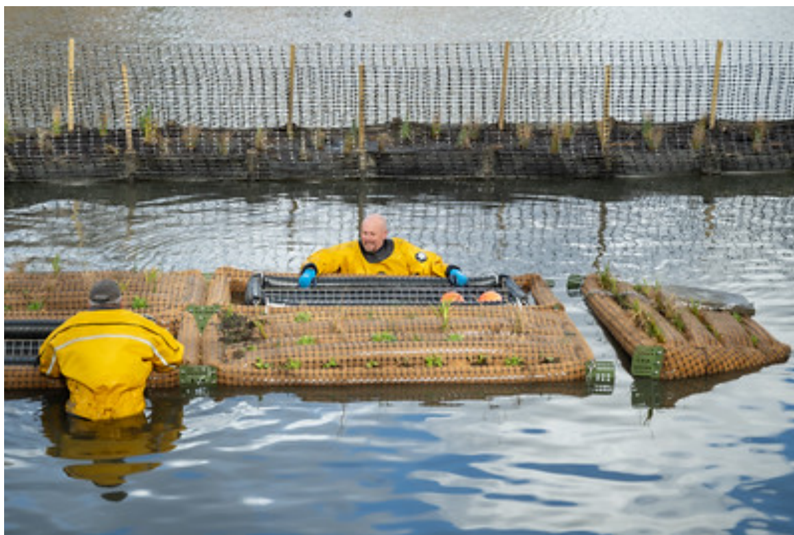
Figure 17: Peabody staff connecting the floating wetland pieces together.
