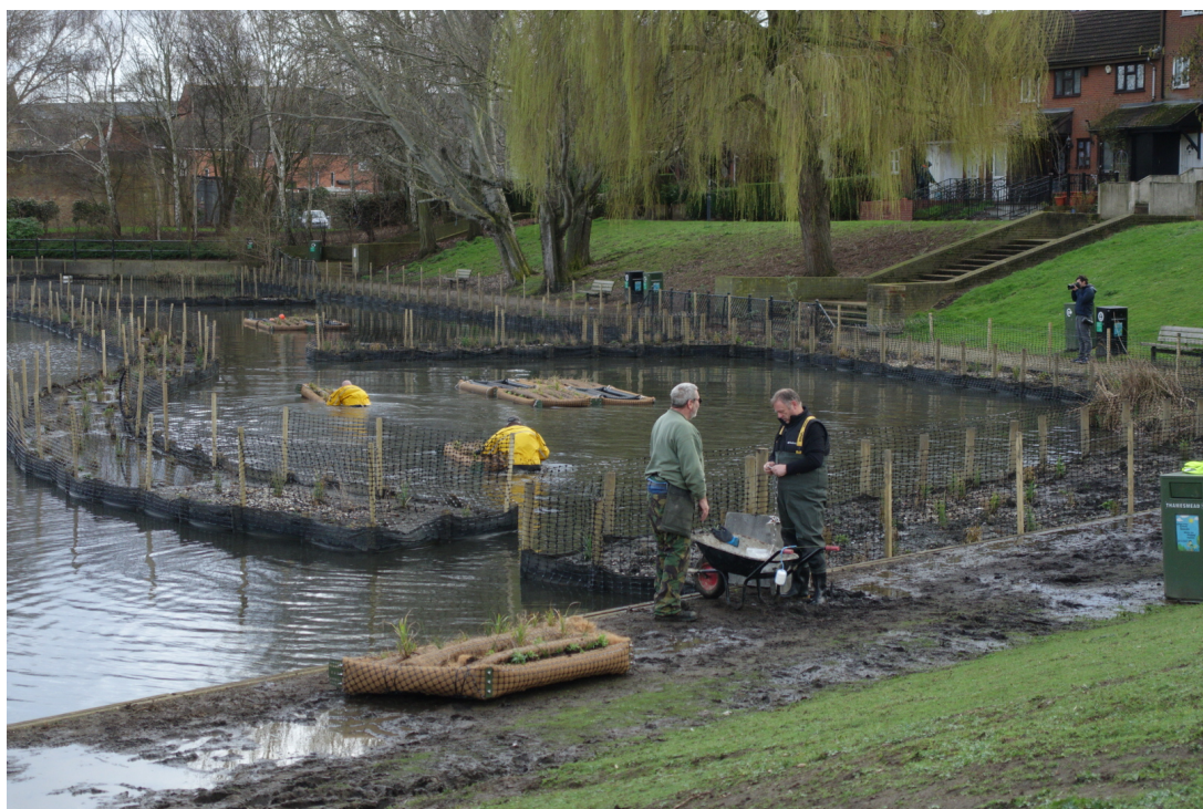
Figure 15: Peabody staff in their dry suits inside Gallions Lake arranging the floating wetlands and connecting them together.
