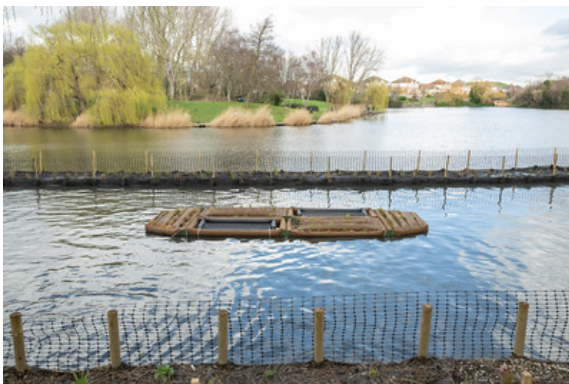
Figure 18: Floating wetland placed within the existing revetment work in Gallions Lake.
